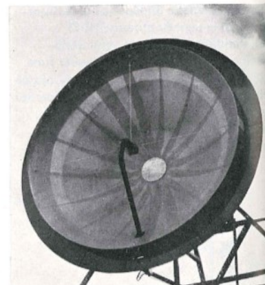
A 4000MHz 10ft diameter aerial
