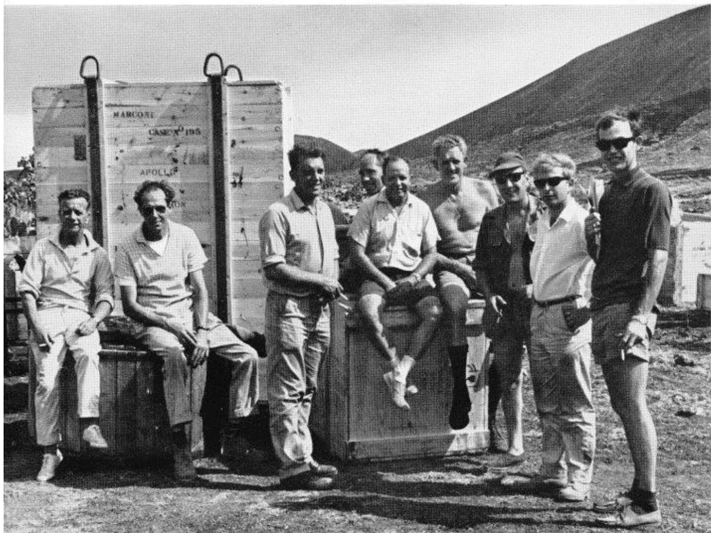
The aerial-erection team—engineers and riggers. Left to right: Johnnie Thompson; Doug Clements; Peter Bowkett; Frank Quinn; Monroe, the American crane-driver; Harry Wilson; Billy Ash; Brian Marjoram, and David Oliver
