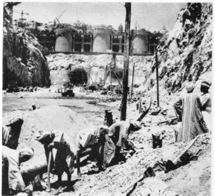
The amount of steel used in the construction of the Aswan High Dam is fifteen times more than that used in the Eiffel Tower. Hewing out the diversional canal was the first stage in the construction of the dam. It was the biggest construction undertaking in Egypt since the Suez Canal [Central Press]
