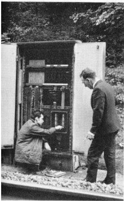
John Carpenter and Hugh Thurgood making a final check of cable connections on the Watford tunnel repeater box
