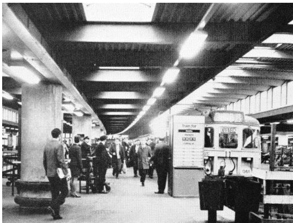
One of the new arrival platforms. Over 30,000 passengers use this terminus daily. There are now 18 platforms altogether, three of which are used for parcels traffic
