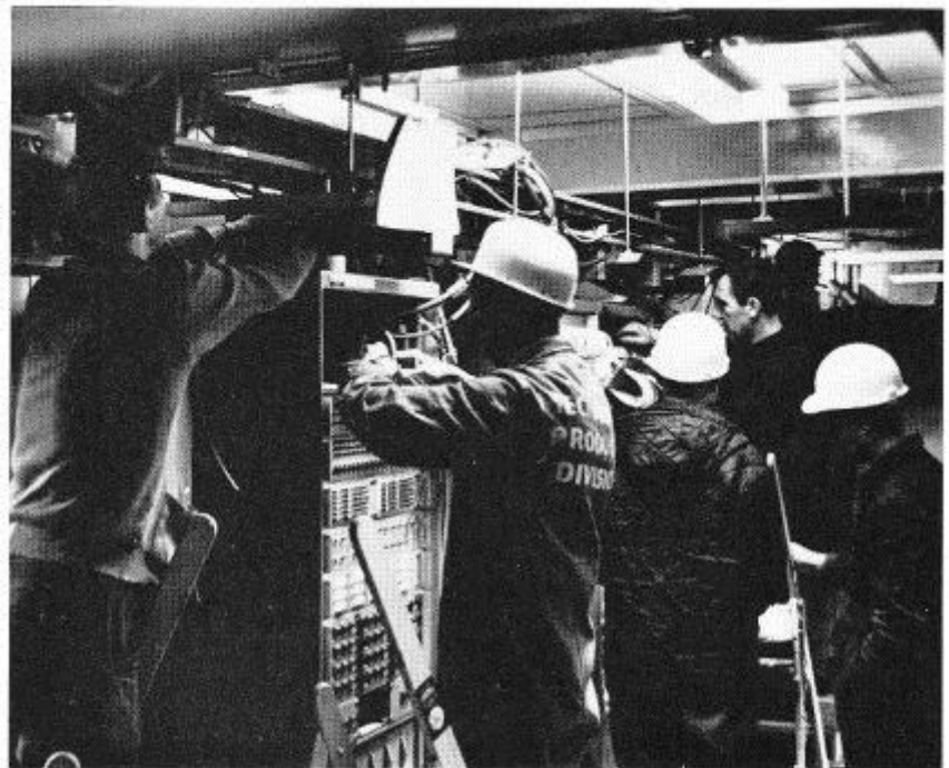
Wiring in progress on the receiver racks. The receiver room is also enclosed within the revolving aerial structure
