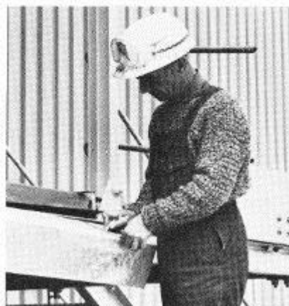
Wiring in progress on the receiver racks. The receiver room is also enclosed within the revolving aerial structure
