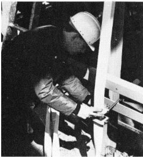
There are four waveguide-runs between the reflector and the transmitters and receivers. Working on them here is Brian Mills who assembled them
