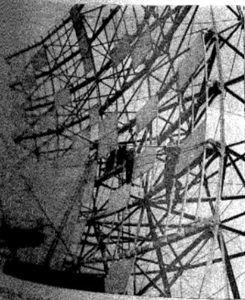
120 ft dish in course of erection
