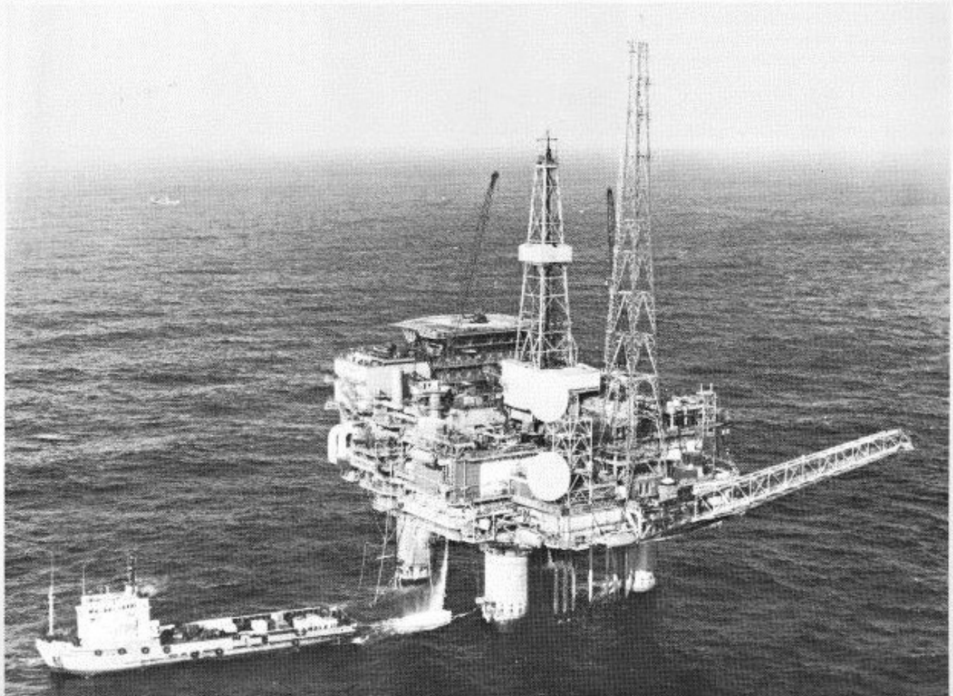
Cormorant oil production platform showing Marconi tropo antennas
