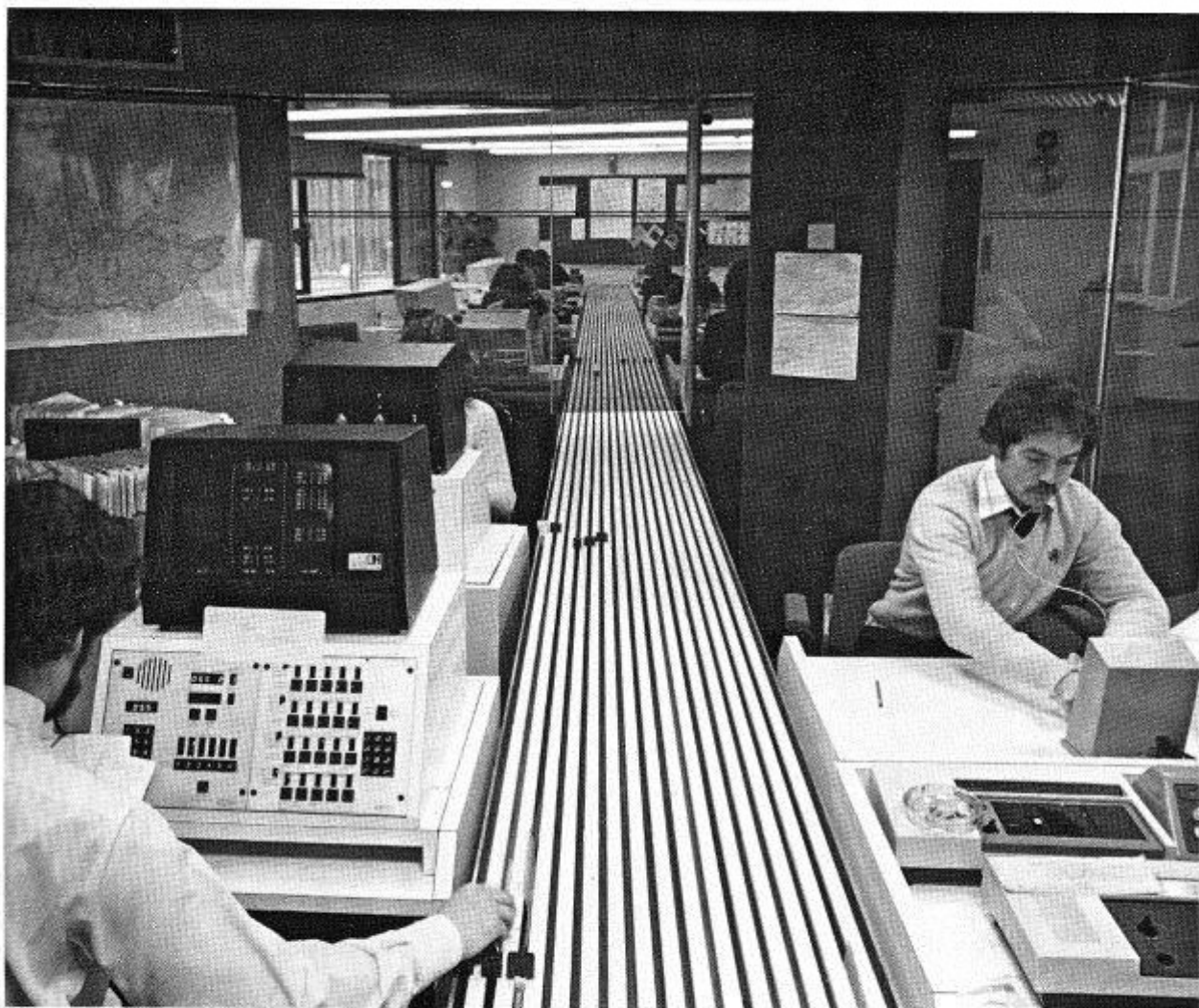
Part of the control room at Croydon
