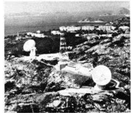
The two Marconi-built antennas at Stanley Point
