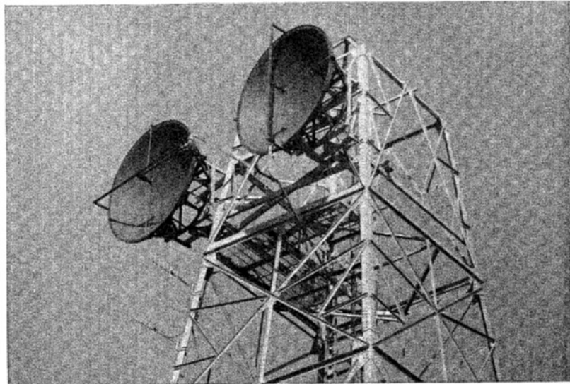
10 ft paraboloidal aerials.
