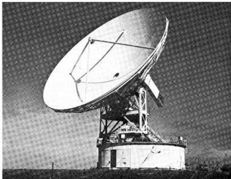
Goonhilly - The highly efficient cassegrain antenna with 19 metre reflector
