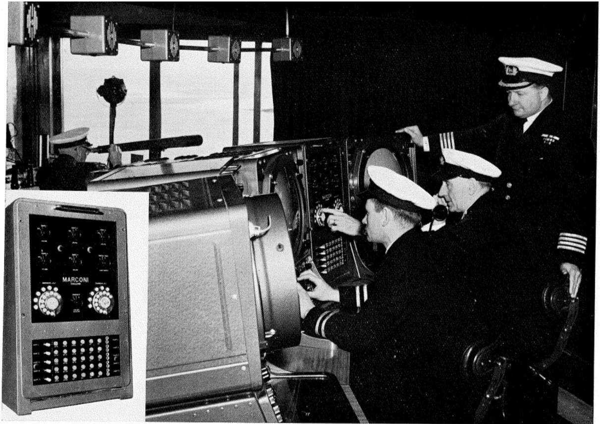
The operating room of Calshot signal station, showing some of the special VHF Radiotelephone equipment installed by Marconi's as part of the Southampton Harbour Board's Port Operation and Information service.
