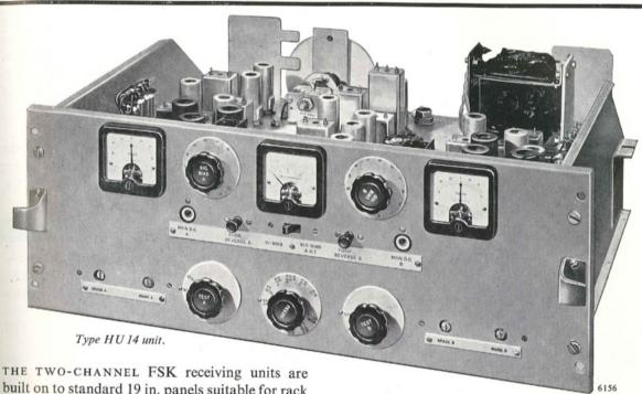
THE TWO-CHANNEL FSK receiving units are built on to standard 19 in. panels suitable for rack or cabinet mounting. The Type HU 14 is designed for fitting into Marconi diversity equipment Type HR 91, while the Type HU 14A is intended for use with the Types HR 11 and HR 13 receivers. The Type HU 14B unit is intended for adapting existing installations of Type CRD 150/22 equipment to diplex reception.
