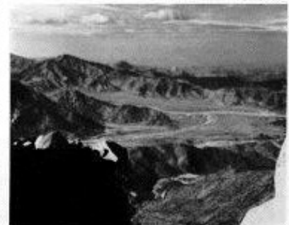
'The road from Jeddah to Riyadh in the Al Hoda Mountains'
