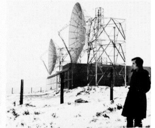
Above: The complete shore terminal at Brummond Hill, near Aberdeen, of the link to the Forties Field. Peter Rackham of Publicity had an uncomfortable journey when he accompanied the photographer to this bleak site. This tropospheric scatter link carries all operating data and other information to and from the production rig 200 miles out in the North Sea.
