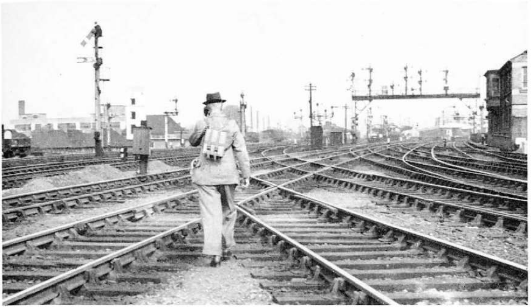
A Railways supervisory engineer in touch with the signal box saves hours of time when men are working on the line
