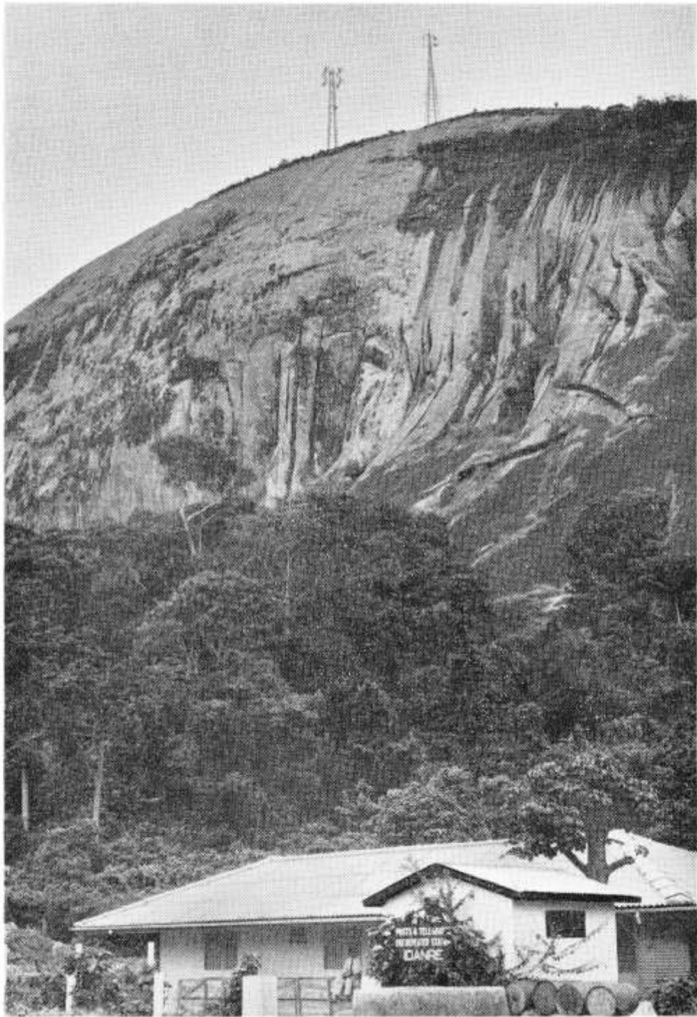
Idanre repeater site. The diesel generators are located at the foot of this 750 ft crag for ease of access; the radio equipment is installed adjacent to the aerials, access to which has to be on foot
