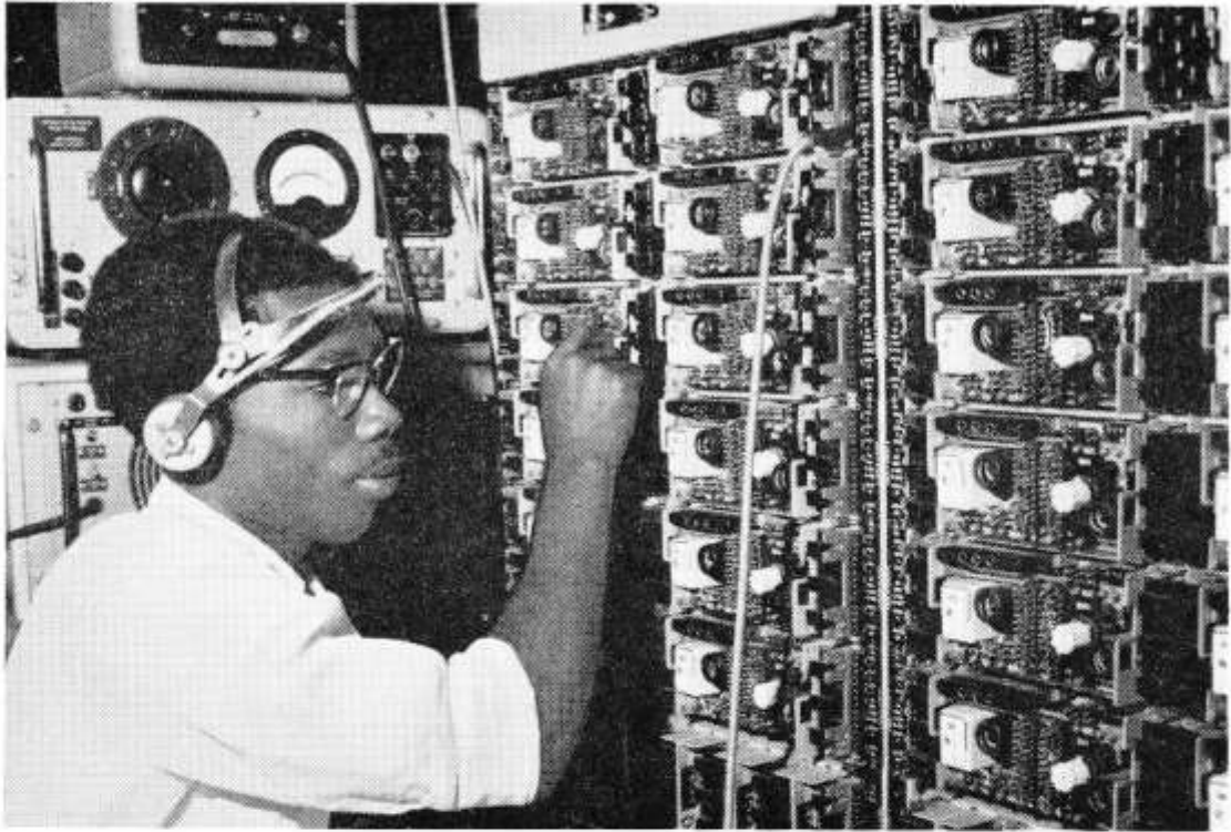
Adjustment to channel panels, Lagos
